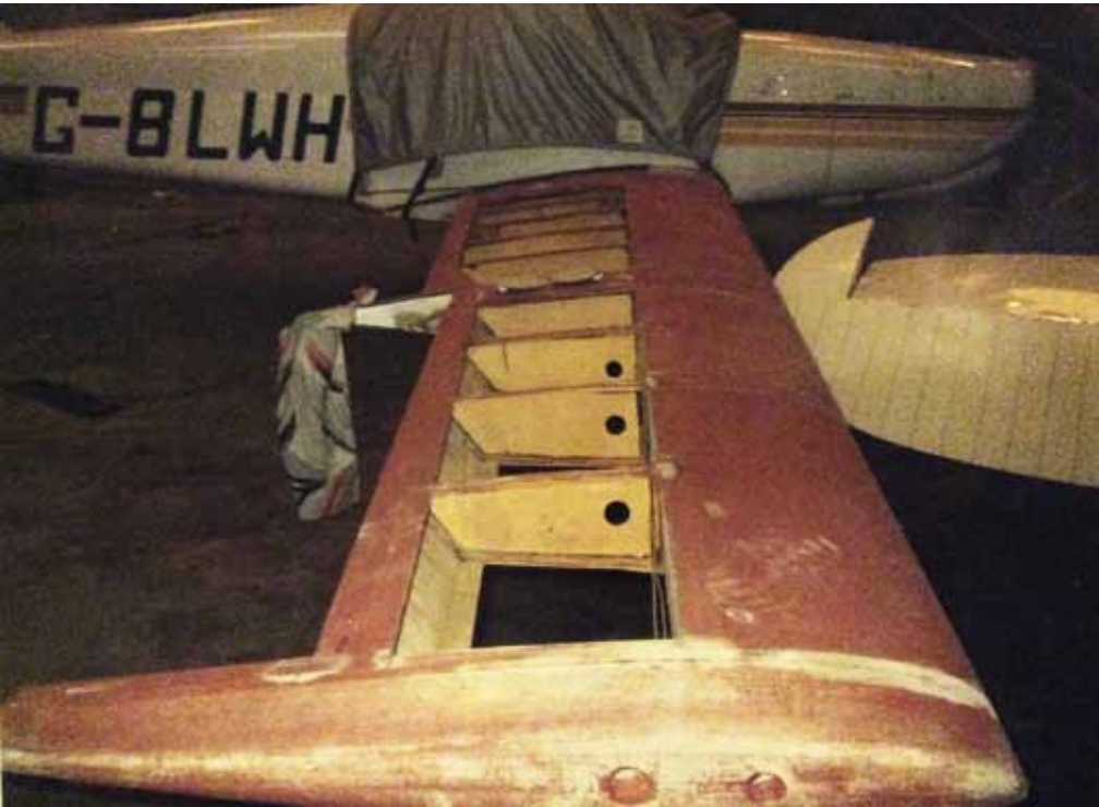
Fuzzy snaps bear witness to previous minor repairs to Whisky Hotel's wing woodwork...
